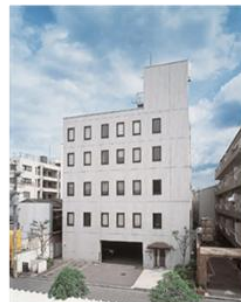
Newly built and opened Data Processing Center (now Head Office)(1989)
