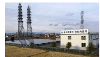
Installed solar power at KUSATSU FA Center(2014)
