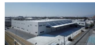
Opened Osaka Distribution Center(2019)
